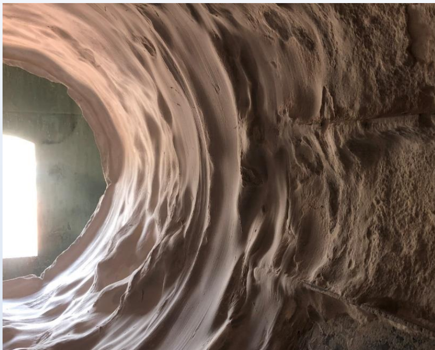
Scale build-up inside kiln
